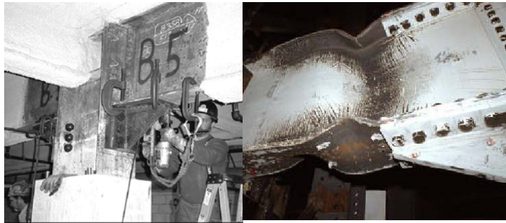
Figure 10: ICF Kaiser bolted connection and test
